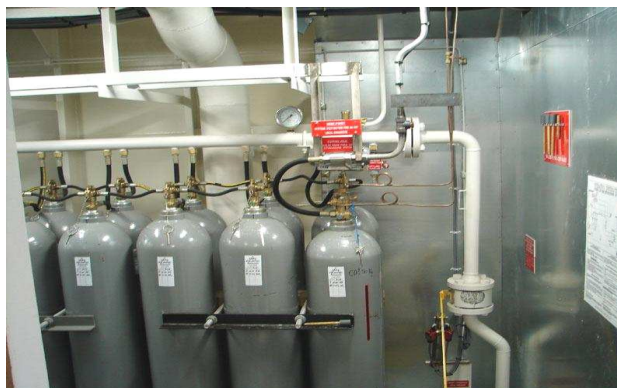
Illustration 7: CO 2 gas pressure system
