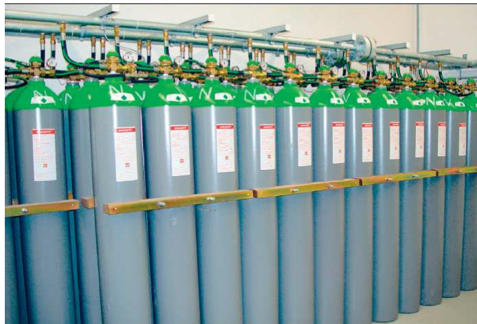
Illustration 8: Group of extinguishing gas bottles, nitrogen
