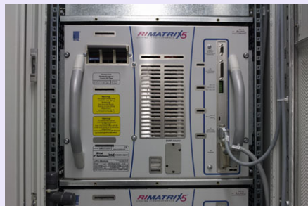
Three-phase, modular "n+1"-redundant UPS technology for secure power on demand.
