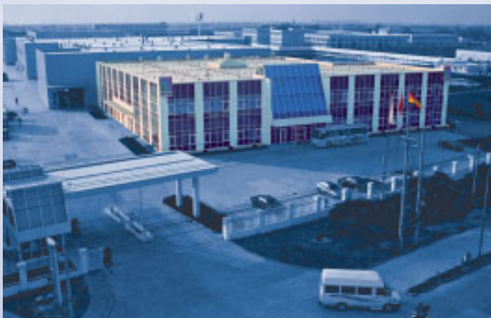
Rittal Electronic Systems: Centre of excellence in Shanghai
