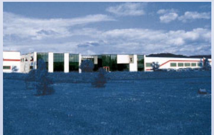
Rittal Electronic Systems: Centre of excellence at Ertop, Joigny
